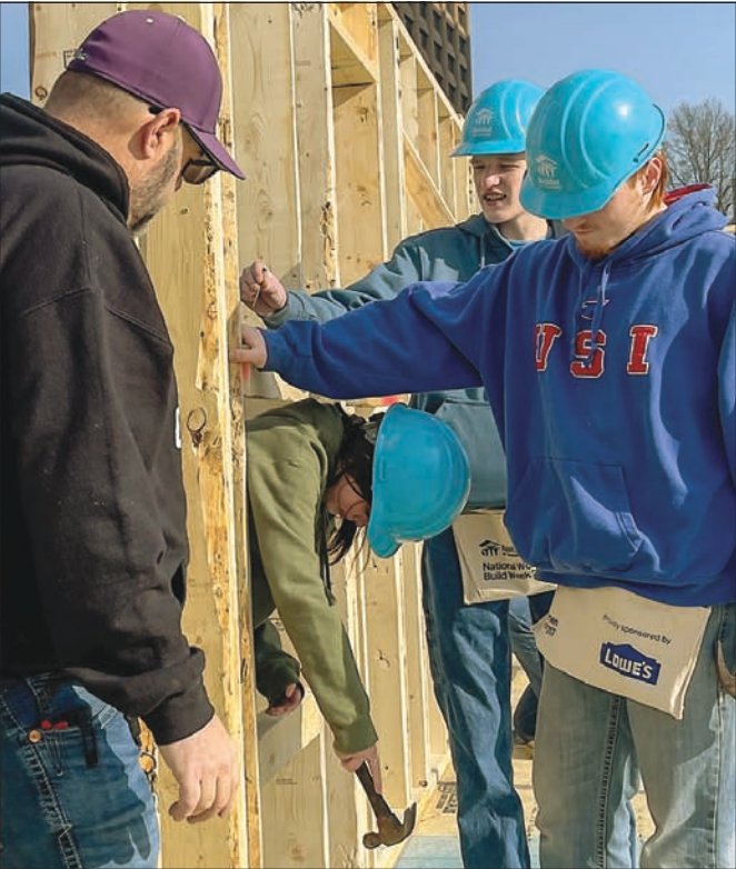
Shown from left are Gilmer High School Construction teacher BJ Chancey, Alivia Richards, Clint Carver and Cole Bolinger.
