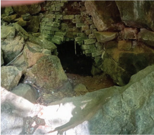
A collapsed wall reveals the inner area of the shaft where limestone was burned
