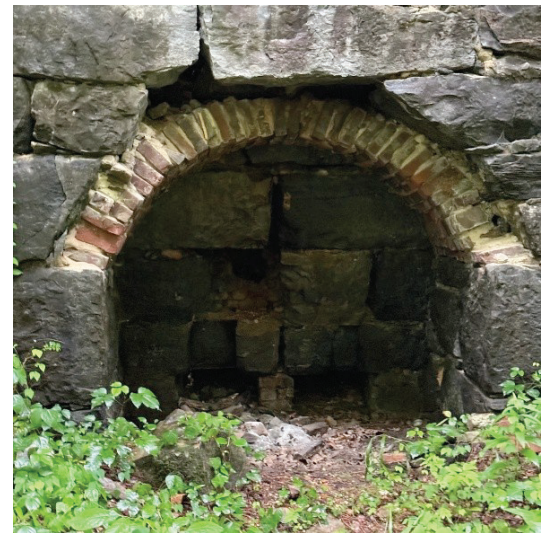
Beneath this arch is where the quicklime would be extracted
