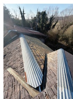
So, repairs made using an existing inventory of wooden shingles!
