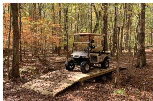
New bridge constructed on trail
